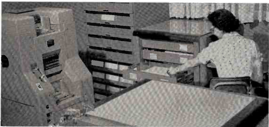
BELOW: This view shows the alphabetical punch that accommodates variable or temporary information by punching holes in cards, and (at left) the collator that assembles several sets of cards into one set in numerical sequence. Checking the file is Olga Slot.
